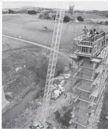
Above: Concreting of pier top on the west bridge, May 1988. Left: Launching of the bridge deck near completion, with the deck about to land on the fifth pier. Below: Construction of piers for the Bendigo-bound carriageway.
