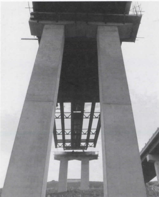
Above: Concreting of pier top on the west bridge, May 1988. Left: Launching of the bridge deck near completion, with the deck about to land on the fifth pier. Below: Construction of piers for the Bendigo-bound carriageway.
