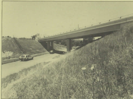
Bridge carrying Kempston Street over the Bypass
