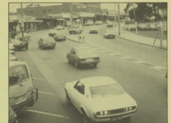
The purpose of the Bypass is to remove through traffic from Greensborough's commercial centre.
