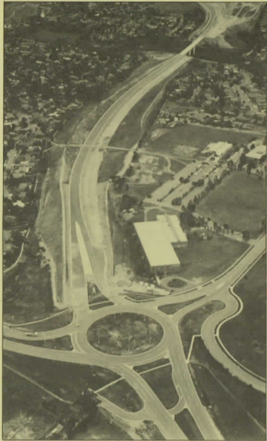
Aerial view showing roundabout at Diamond Creek Road
