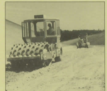
Earthworks on the project
