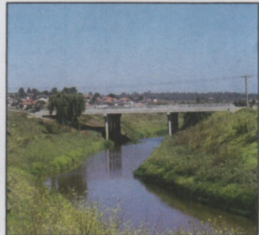
Wallis Creek bridge.
