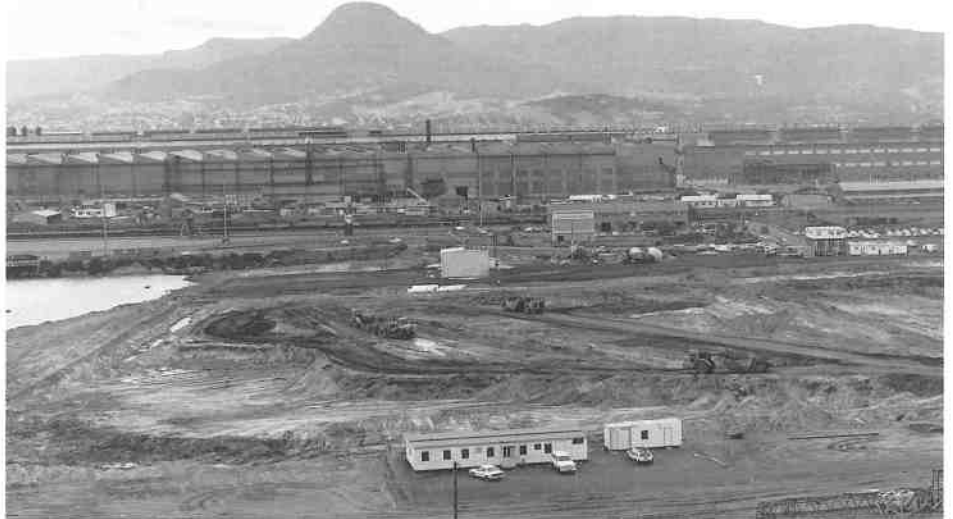
The Tunnel casting basin at Port Kembla
