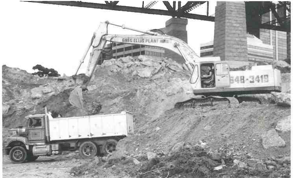
Work in progress in Bradfield Park, Milsons Point for the Tunnel
