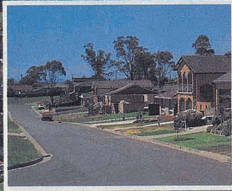
Proper planning and new major works leave residential areas free of through traffic.
