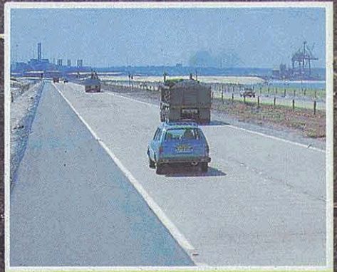
Commercial and industrial activity needs good roads.
