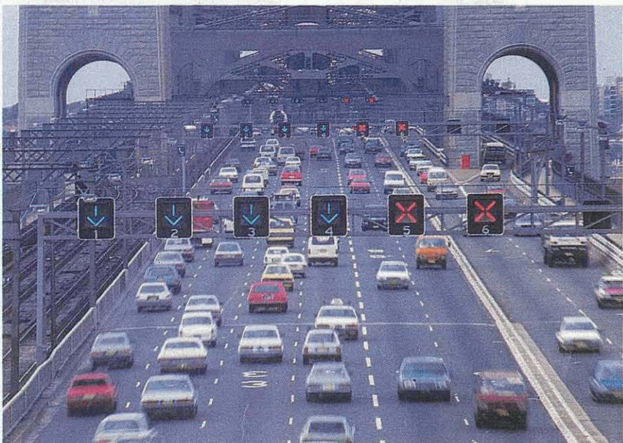
Electronic lane control on the Sydney Harbour Bridge was introduced to improve traffic flow over Australia's busiest section of road.
