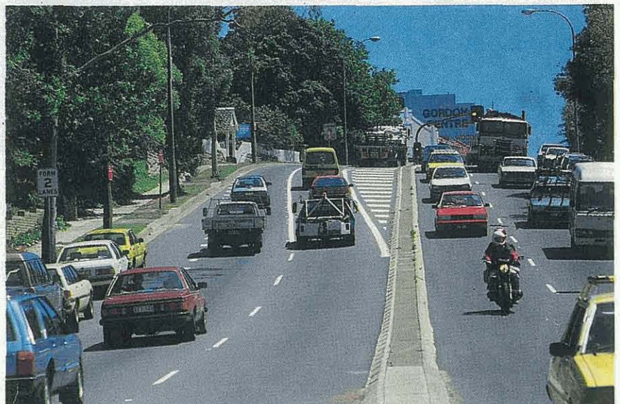
S-lanes allow vehicles to await a right turn without disrupting traffic flow.
