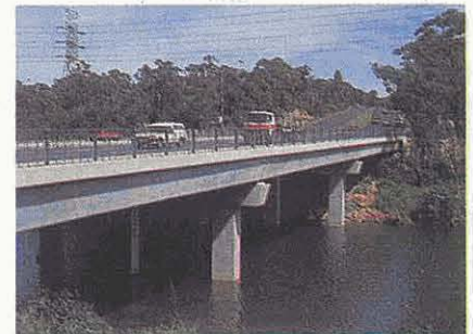
Duplication of the bridge over Lane Cove River has eased congestion on Epping Road.
