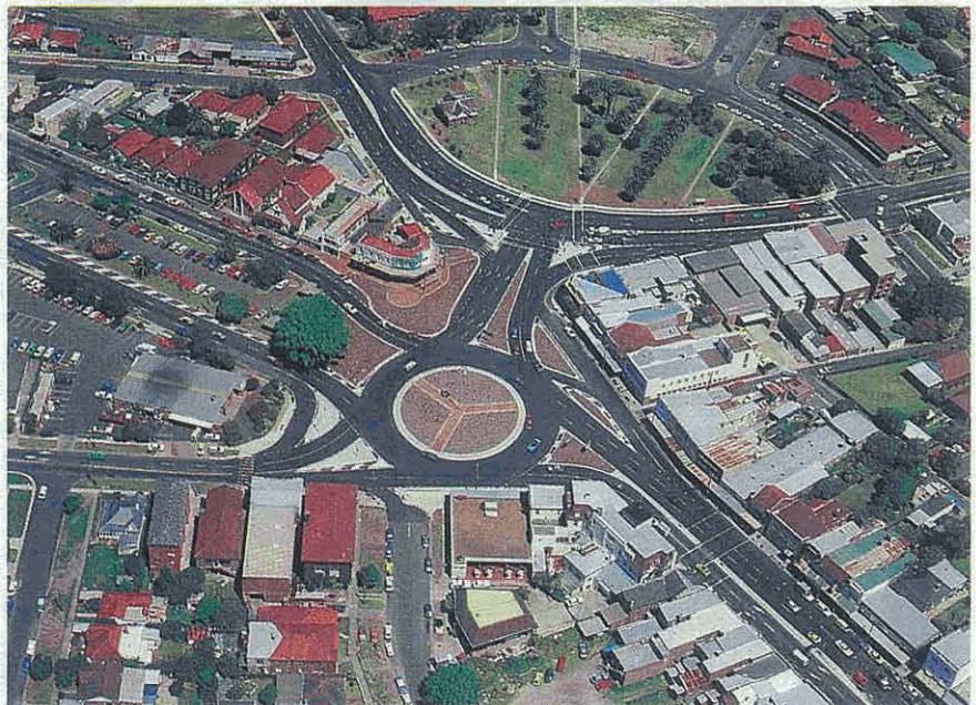
Reconstruction of the roundabout at the intersection of Bunnerong and Gardeners Roads, Kingsford, has removed the intersection from the Accident Blackspot List.
