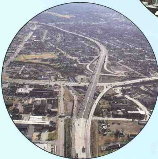
Completion of the F4 viaduct means uninterrupted freeway conditions from Concord to Mays Hill.
