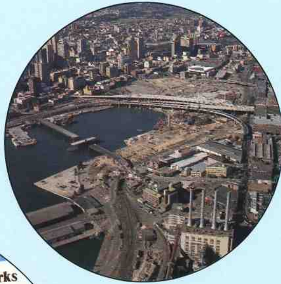
Work progressing on the Darling Harbour viaducts to White Bay.
