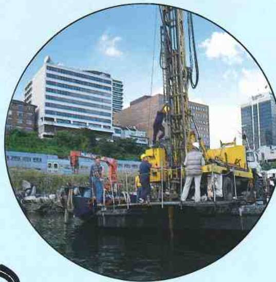
Test drilling in progress for the Sydney Harbour Tunnel project.
